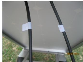
Illustration 3: NEGATIVE (-) is on the LEFT. POSITIVE (+) is on the RIGHT.
