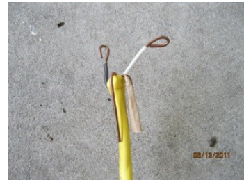
Illustration 11: Stripped electrical wire with looped ends. Note that the ground wire is folded out of the way.
